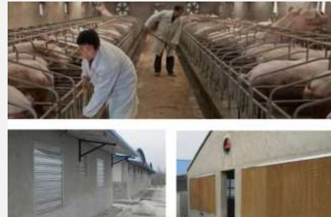
Swine farm exhaust fan 养猪场通风
