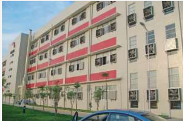
Commercial building ventilation 商业建筑通风
